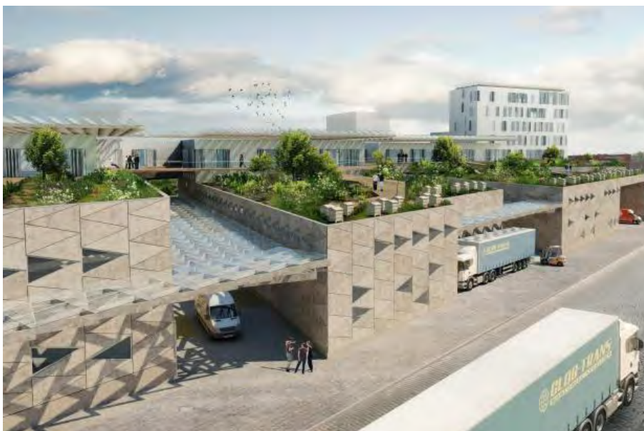
Greenbizz Brussel (bron Wilkinson Eyre Architects &amp; Grant Associates)
