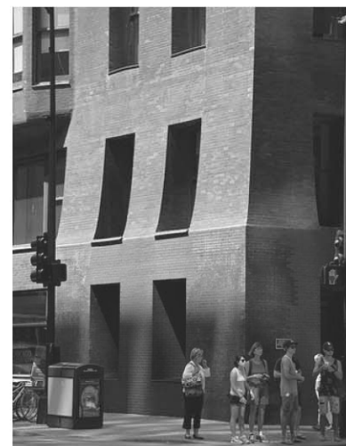
rechts : D. Burnham and J.W Root, Monadnock Building, Chicago, 1890 links : principe van de versmallende gevel
