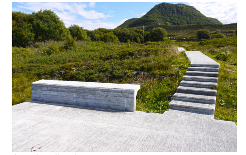
A verharding beton
