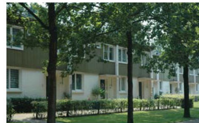
BUREAU LUBBERS, HERSTRUCTURERING WITTE WONINGEN, VENLO (NL), 2008
