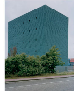
Antwerpen Petrol Substation, noA
