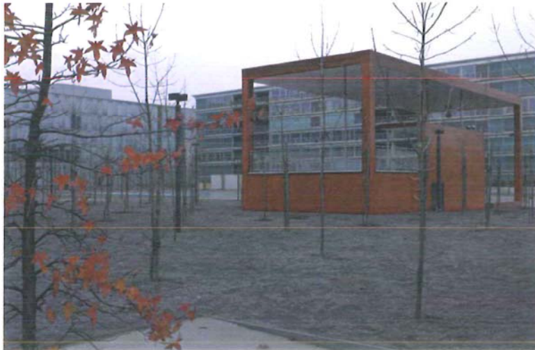
Project Oerliker Park
