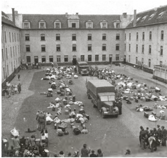
① binnenplein Dossin courtyard Dossin
