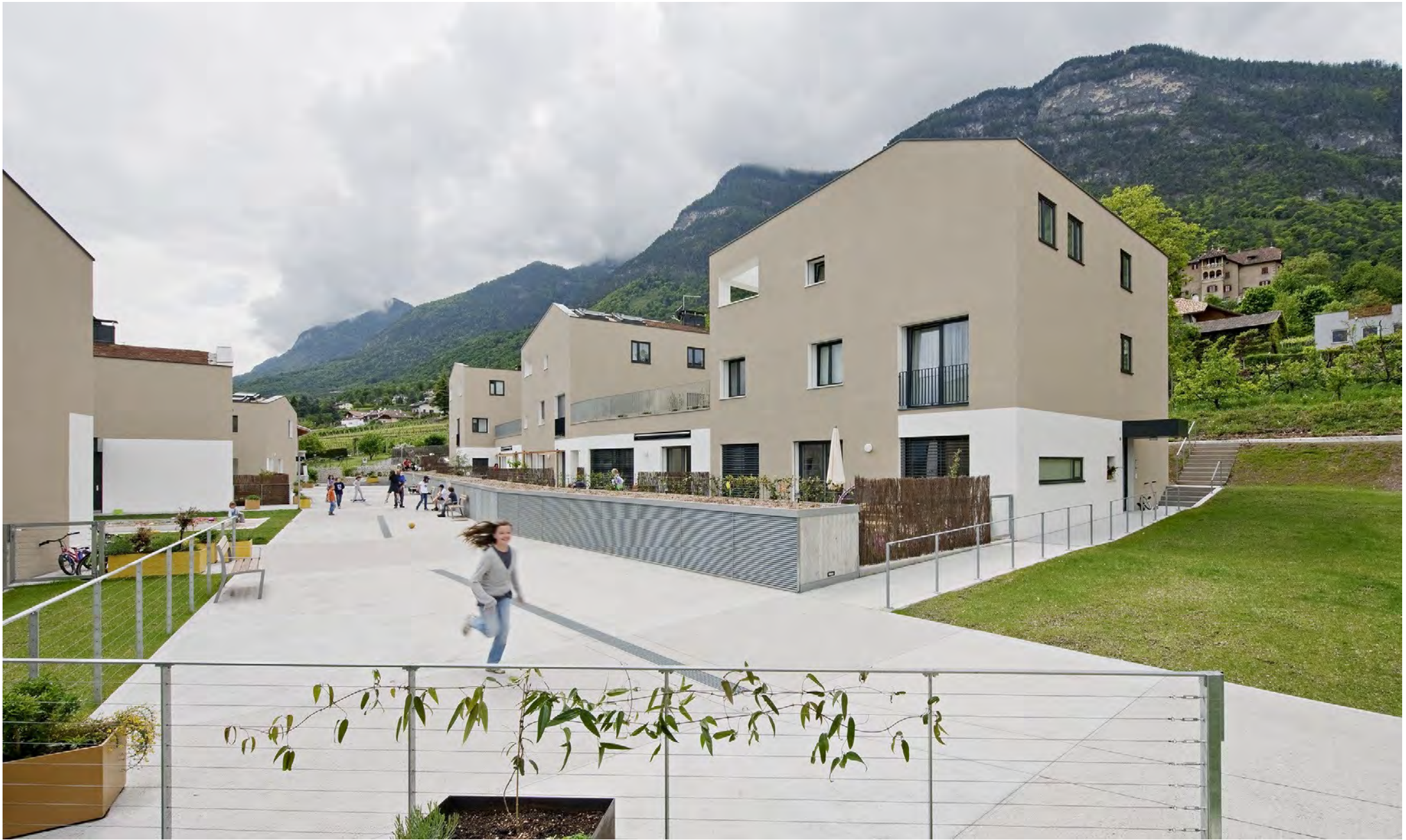
The play street forms the interface between public and private. The ventilation shafts of the underground car park partly mark the border to the private gardens.
