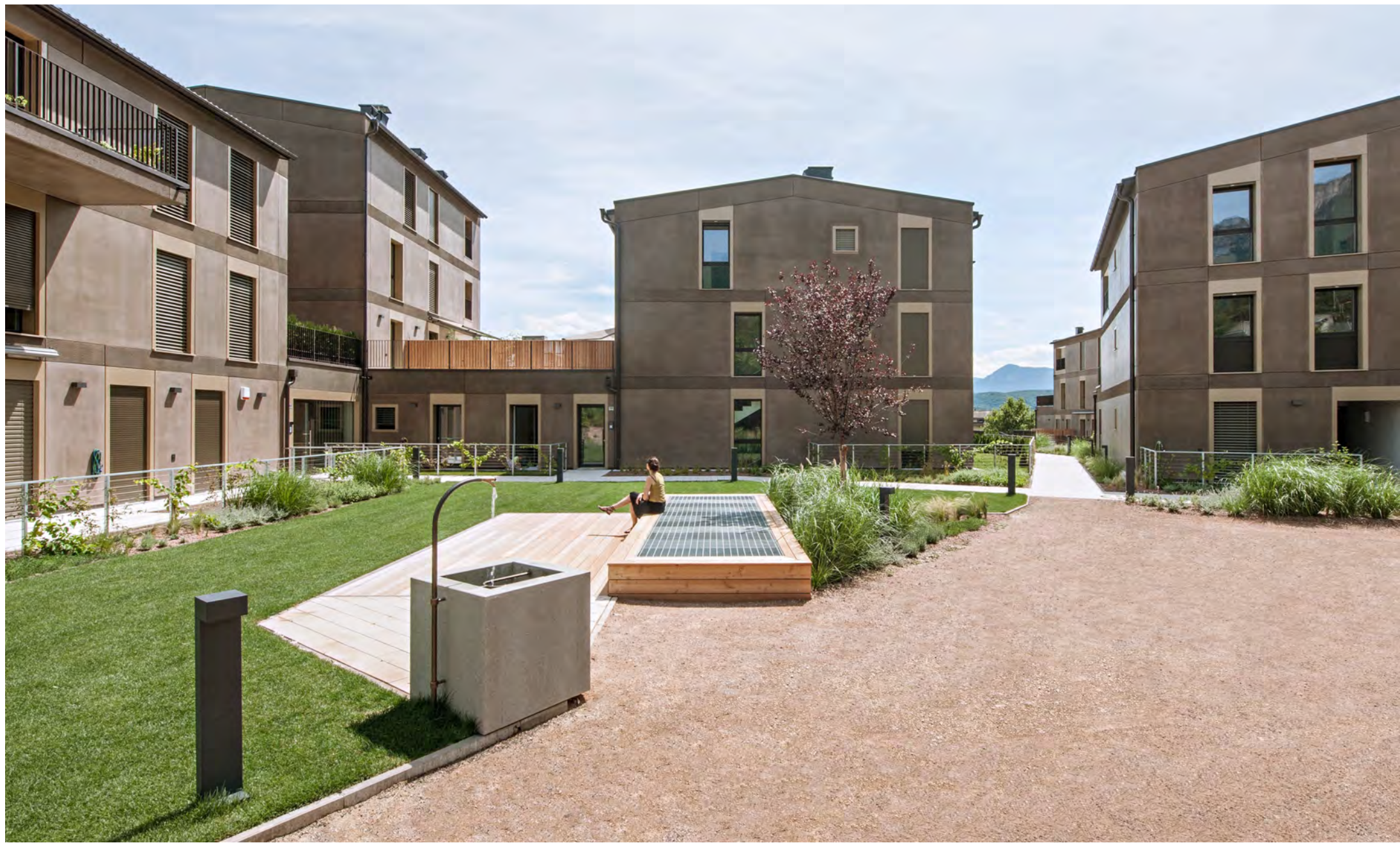
The village green with its fountain, wooden terrace and bench, as well as play areas and footpaths, emphasise outdoor living, which strengthens the sense of community among the residents of the estate.
