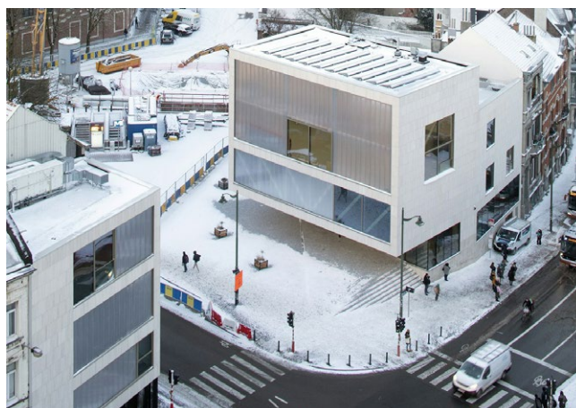
Centr'Al, Brussels, B-Architecten, 2020 © Maxime Delvaux
