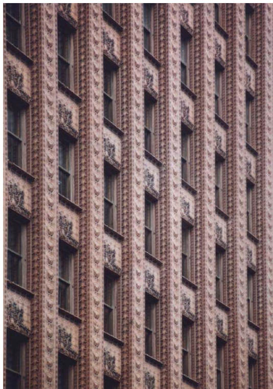
Guaranty Building, Sullivan, Buffalo
