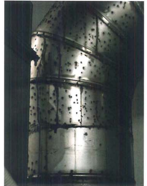
Surface rusting on stainless steel due to corrosive pool atmosphere
