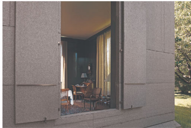
Garden Pavillion Christ en Gantenbein, 2012
