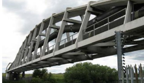
Peston Pipe Bridge - Ingleyby Barwick (UK)
